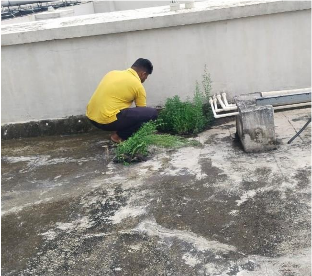
Roof Cleaning on 21.09.2023 in ESIC Hospital, Angul
